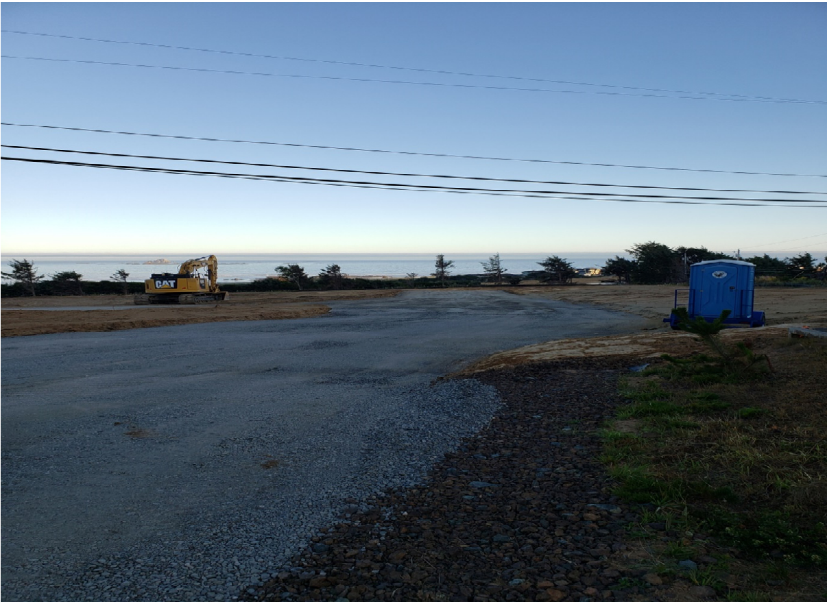
Pacifica at Rogue Reef Subdivision-Existing Site Conditions
